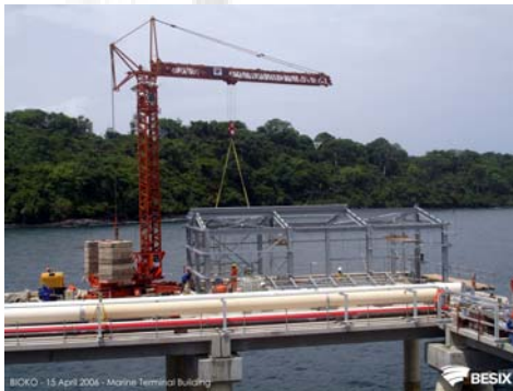
BOKO - 15 April 2006 - Marine Terminal Building
