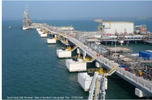
South Hook LNG Terminal - View of the Berth Line at High Tide - 07/05/2008
